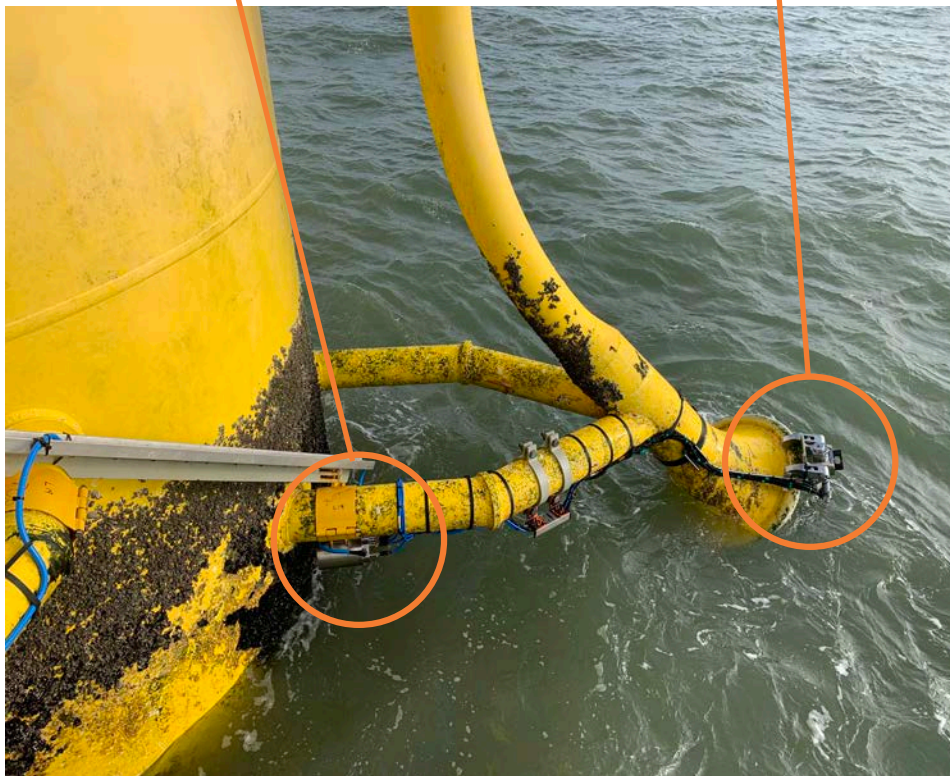
Figure 2: Subsea Enclosure and Load Cells, London Array Wind Farm (Kent, UK)
